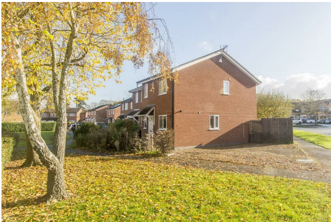
Side Elevation photo
